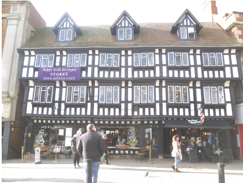
Plate 31 No. 207-210 High Bridge, these grade I listed shops date from C16th, and are the only surviving example of a medieval bridge carrying shops and houses.
