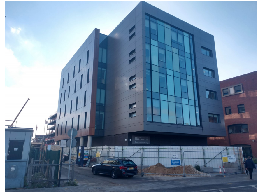
Plate 70 The Sarah Swift Building, Brayford Wharf East, new development within and adjacent to the conservation area should seek to reinforce the historic grain.
