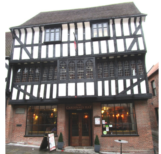
Plate 56 No. 268 High St is a Grade II* listed inn building and dates from the late C15th. It was restored in 1952 and has close studded timber framing and 2 jettied floors.
