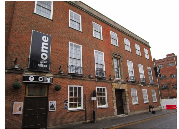
Plate 61 The Annexe, Park St is the former Navy and Air Force Institutes (NAAFI) Club and makes a positive contribution to the conservation area.
