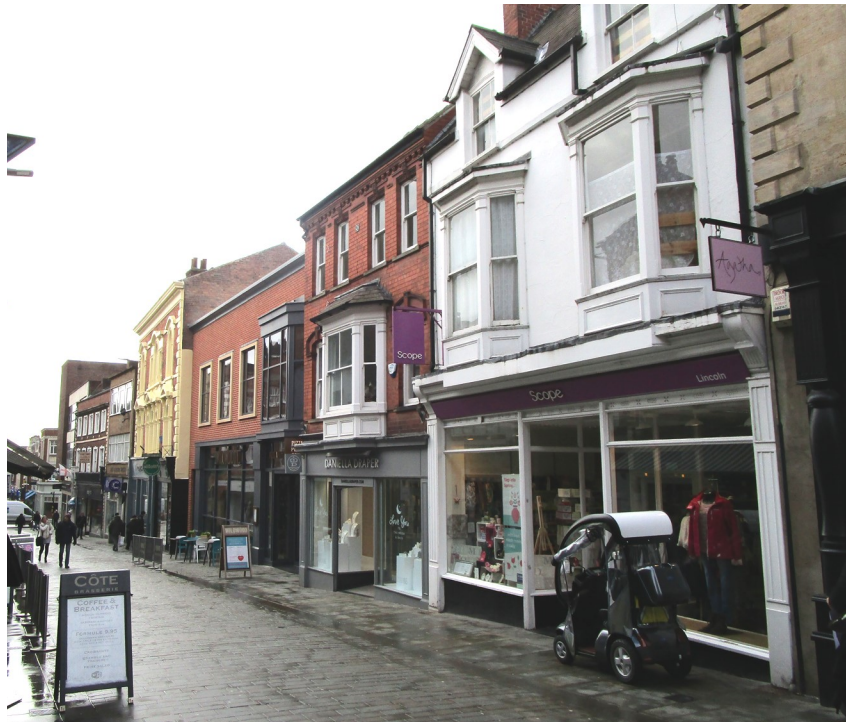
Plate 77 No. 260-261 High St – examples of well- designed shop fronts and signage, with well proportioned, traditional components of a shop front including console brackets, fascia, pilasters, transoms, mullions and stallrisers. Small hanging signs are used to provide projecting signage.
