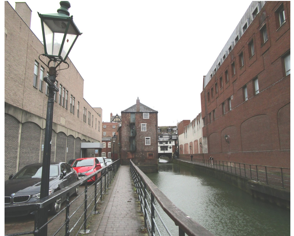
Plate 23 The view of High Bridge from the west is enclosed by large, modern retail units.
