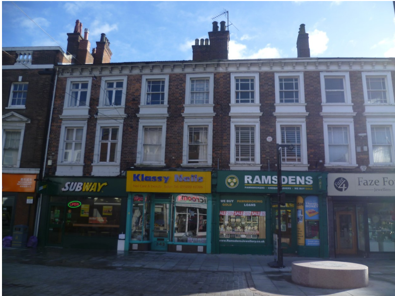
Plate 64 No. 343-345 High St, despite having shop fronts that could be improved, this retains its architectural interest on the upper floors.
