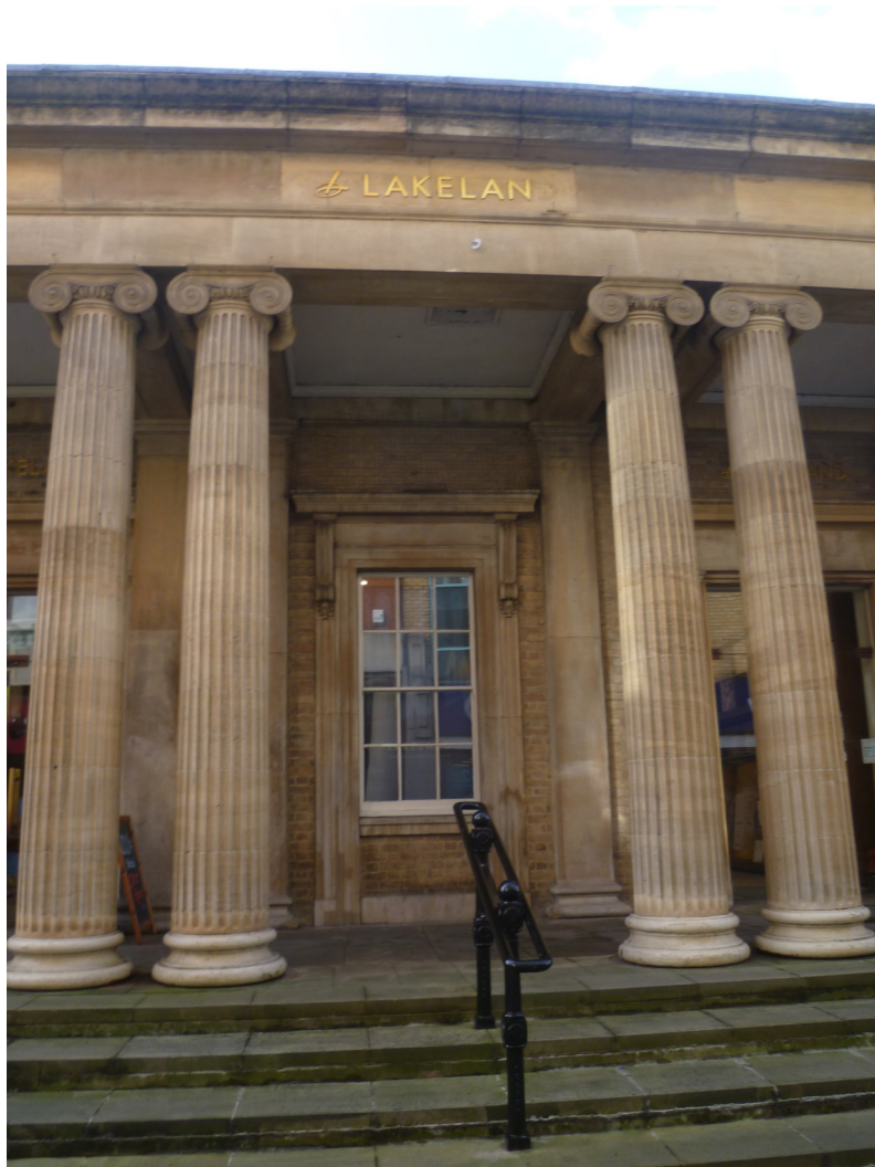
Plate 36 The Ionic columns on the former St Mark's Station, Station St
