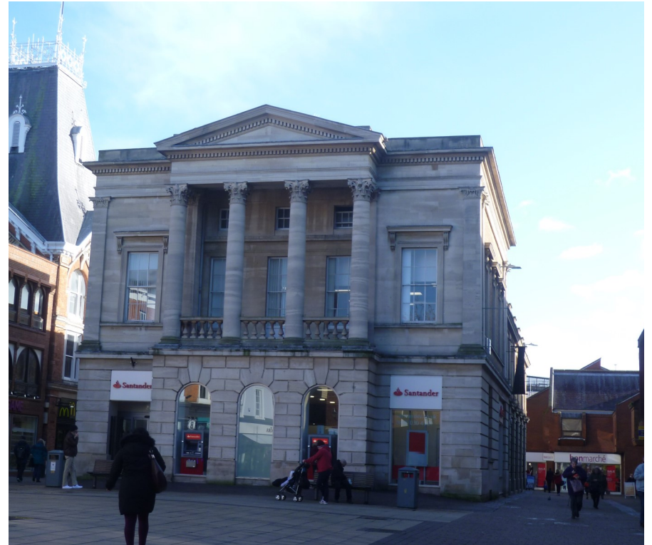
Plate 28 Former Corn Exchange, Cornhill dated 1847 and designed by W A Nicholson, it is dominant within Cornhill.
