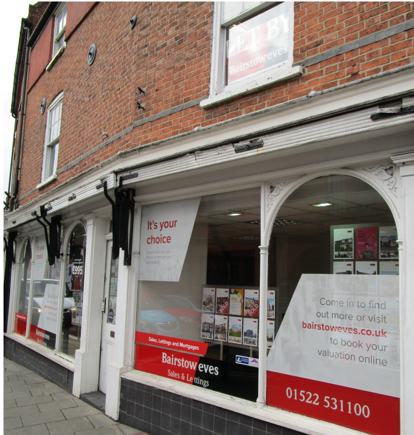
Plate 73 No. 21-23 Silver St, an example of an historic shop front with historic shuttering. Given the lack of a deep fascia for signage, transfers on the shop windows have been used to provide corporate signage.
