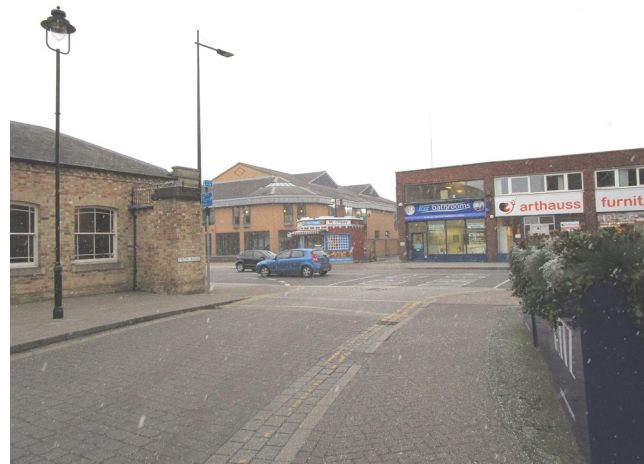
Plate 17 Firth Road showing the former St Marks Station to the left and railway roundhouse to the centre. Behind, the Magistrate's Court has overwritten the former railway landscape.
