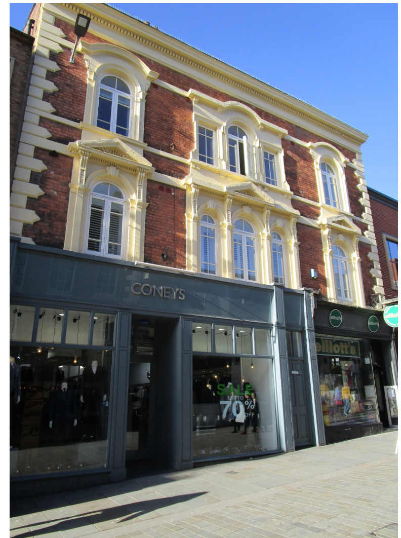
Plate 37 No. 255 High St has decorative stone surrounds to its upper windows, incorporating cill and window head banding, pediments, consoles and dentillation to the 1 st floor, and a Venetian window to the 2 nd . It also displays chamfered quoins, dentilled eaves, and a moulded cornice.
