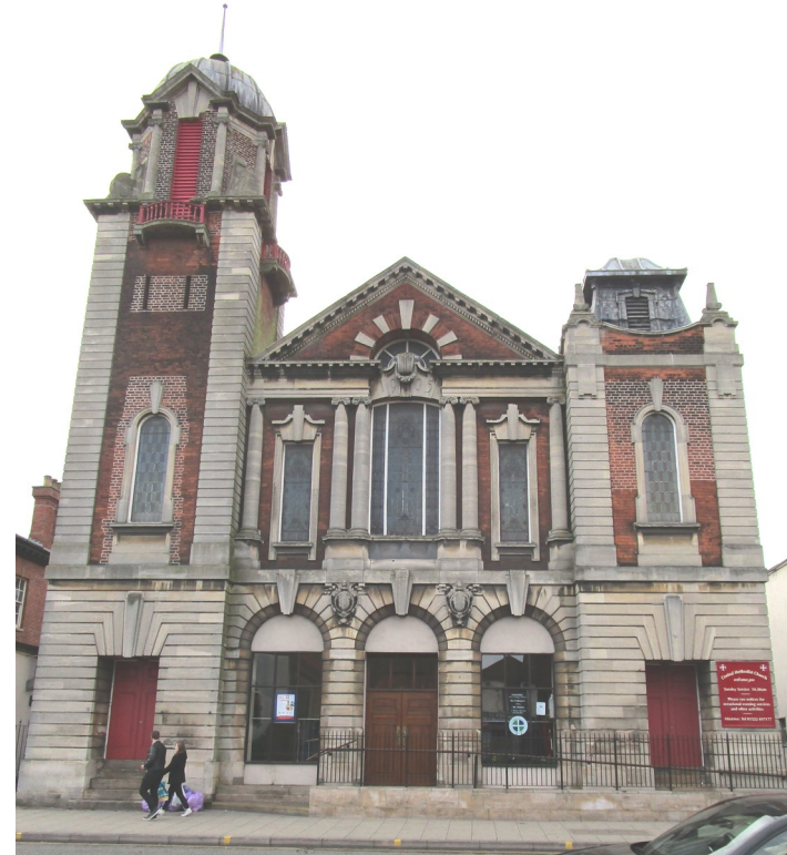
Plate 50 Central Methodist Church, High St is a key landmark within the area with its imposing form and square bell tower topped with an octagonal turret, spherical lead dome and finial.
