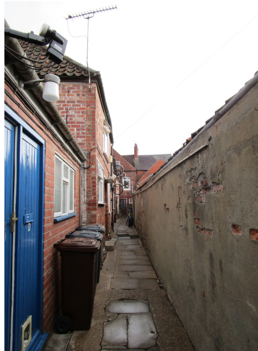
Plate 19 Development at the rear of the burgage plot, 41 Hungate
