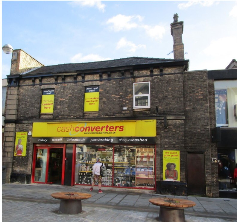
Plate 62 No. 332 High St is part of the former railway stables which formed a much larger complex here. It has architectural and historic interest despite having a poor shopfront and signage.
