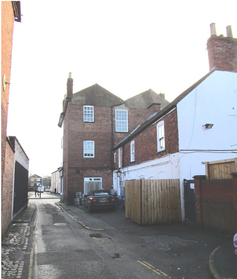
Plate 47 The view of The Anchor pub from Tanners Lane reveals the less altered rear of the building, with 6 over 6 flush sash windows with segmental brick arched heads.
