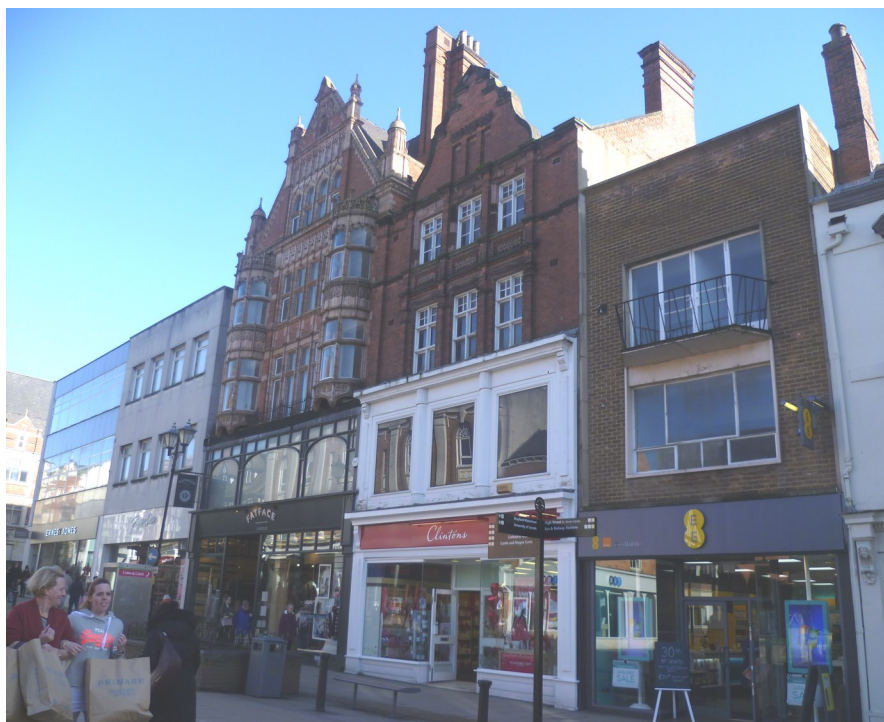
Plate 24 No. 303-309 High St, showing decorative late C19th buildings (centre), indiscriminate modern buildings (left), and the unaltered upper floors of a 1950's/60's building (right)
